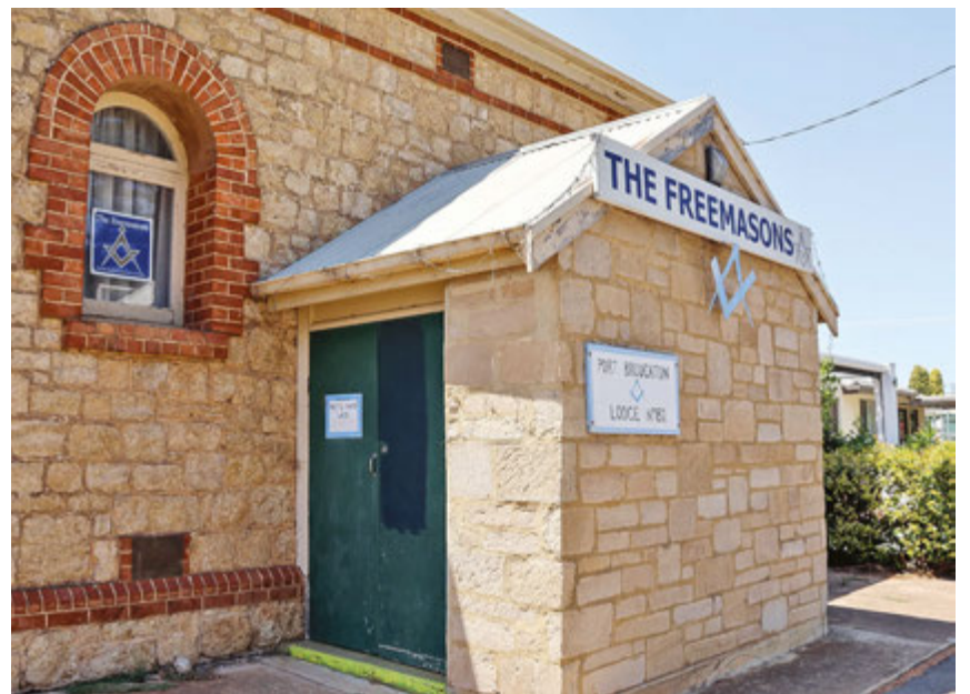
LODGE... The Port Broughton Masonic Lodge.
